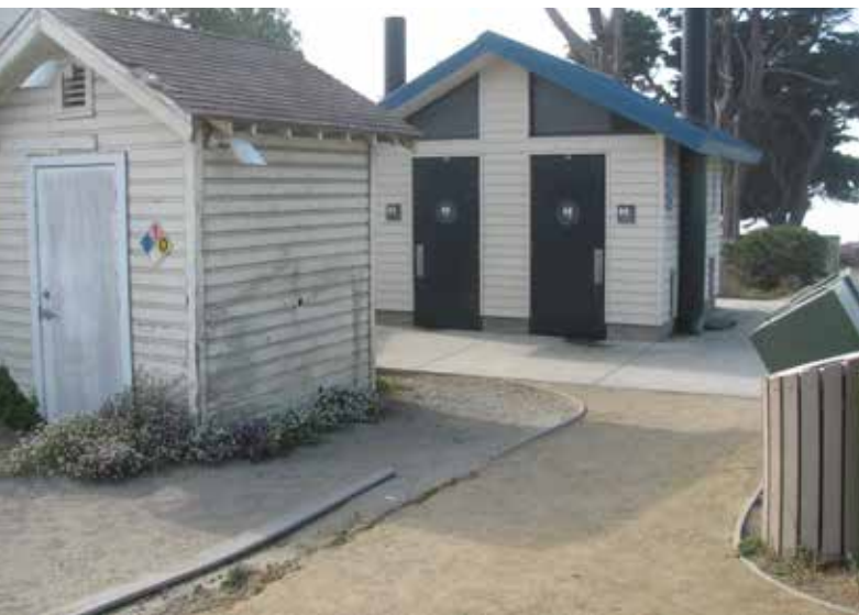
Decomposed granite paving in front of restrooms.
